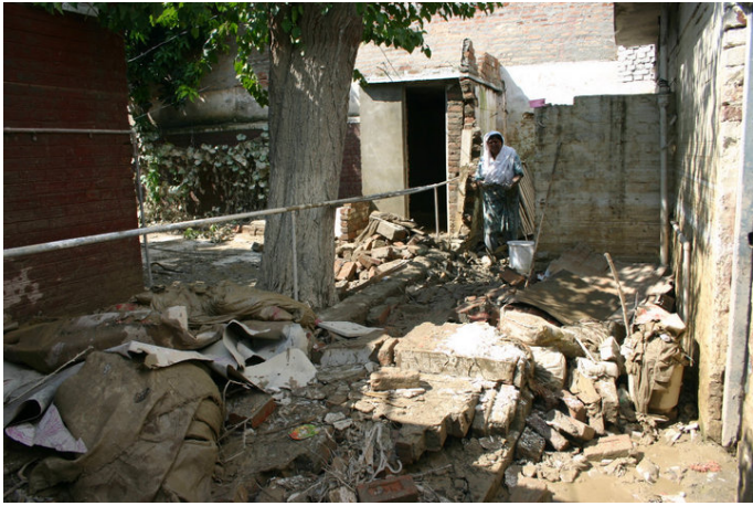
Houses, security walls, and floors are completely destroyed.
